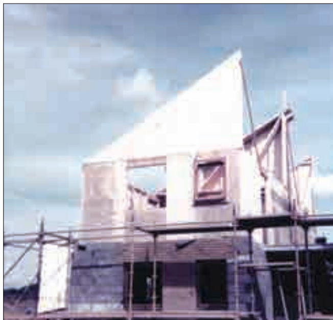
Barratt Solo flats under construction. Image courtesy of Elizabeth Henderson.
