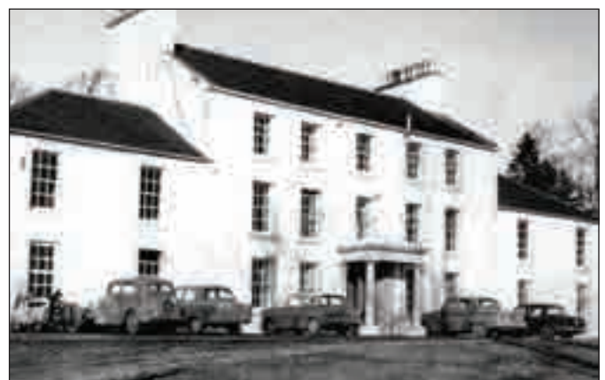
Howden House as Scottish Station of the National Institute for Agricultural Engineering. Image courtesy of Mr Phil Hutchison via WLLHL.
