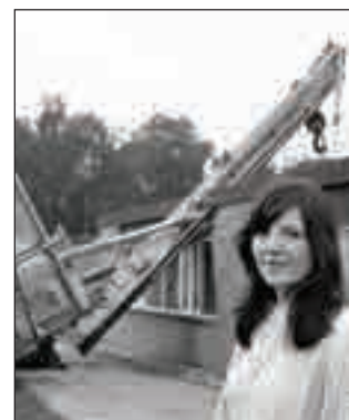
Crane incident at Harrysmuir Primary School. Image courtesy of Johnston Press plc.
