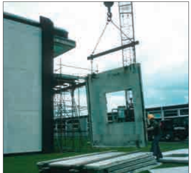
Jespersion housing under construction, c1966.
