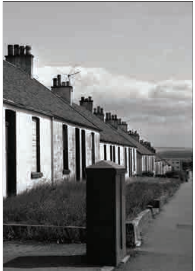
Miners' Rows at Livingston Station, 1970. Housing at Deans South can be seen in the background. Image courtesy of Johnston Press plc.
