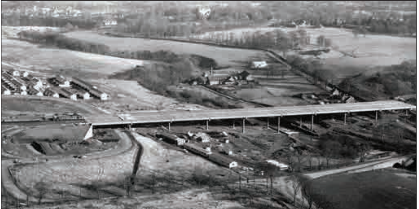
Aerial of Almond Valley Bridge Construction, 1971.
