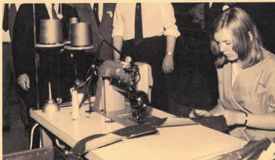
Back pockets whizzing through the hemming machine one after another.
