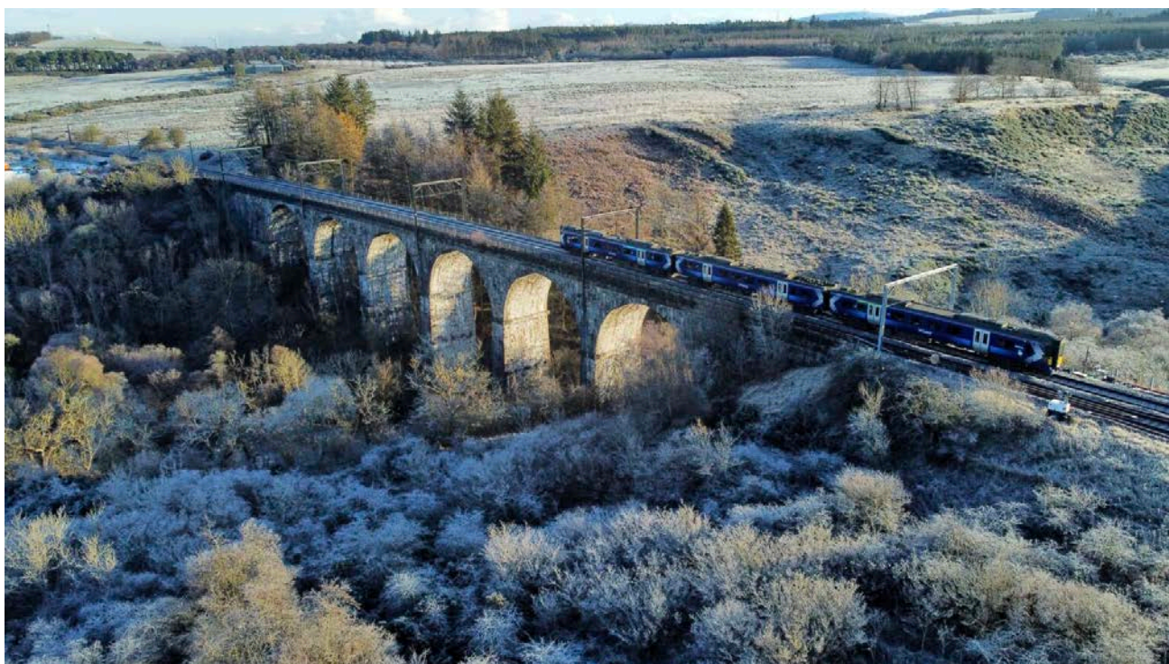
Murieston Community Development Trust / Linhouse Water Railway Viaduct
