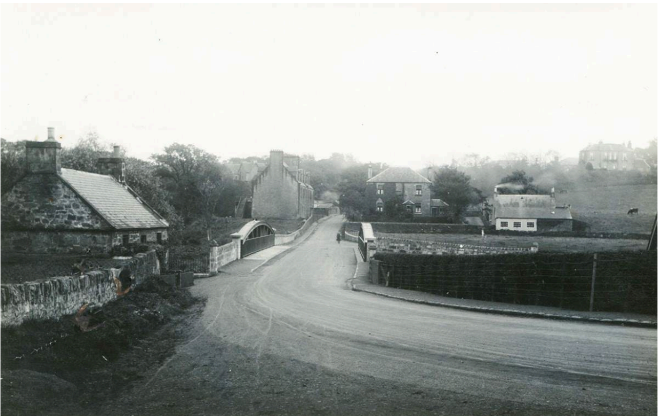
Figure 15: Mid Calder North Bridge 1929. Source and Photo Credit: Scottish Shale 5
