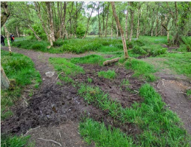
Figure 1 - Drainage issues leading to path braiding and widening
