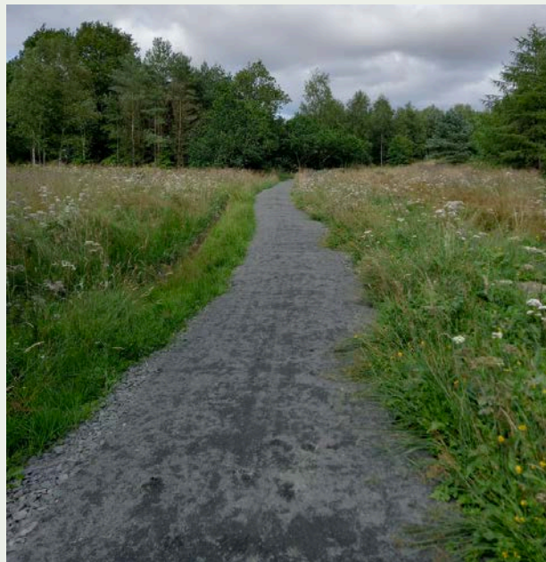
Figure 3 - Example of a type 1 stone path
