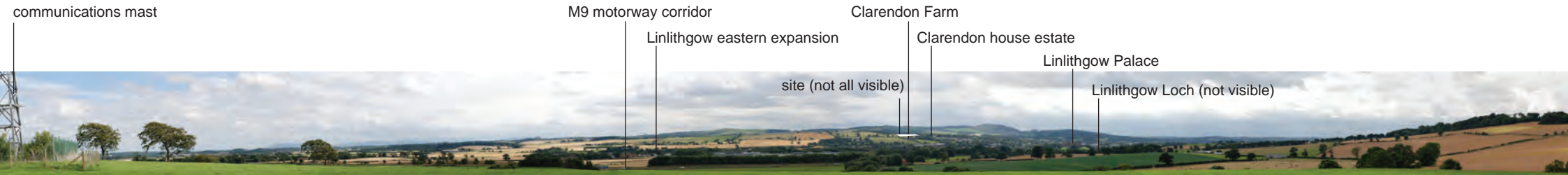
12. View looking south towards the development site over the Linlithgow valley, viewpoint taken at the mast compound at OS Grid Reference NT 015 788.
