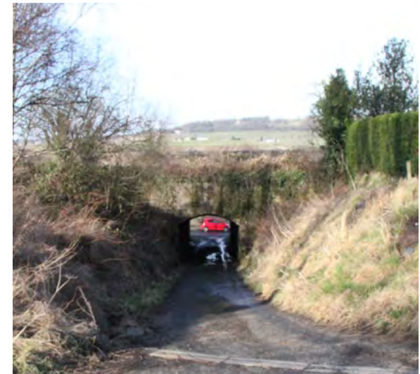
View B - Staney Road, tunnel under Union Canal
