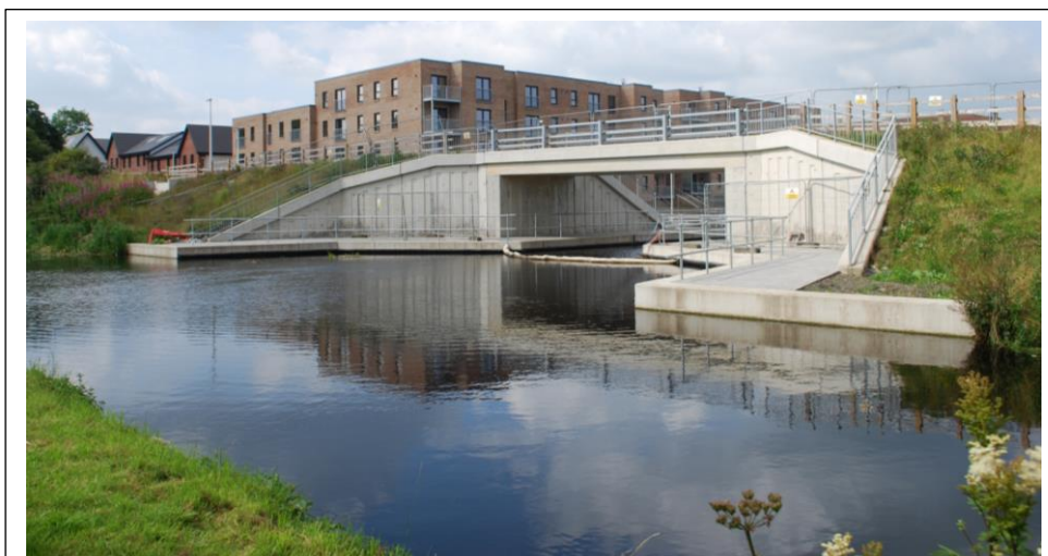
Photo 2. Marina bridge 32b canal side view
