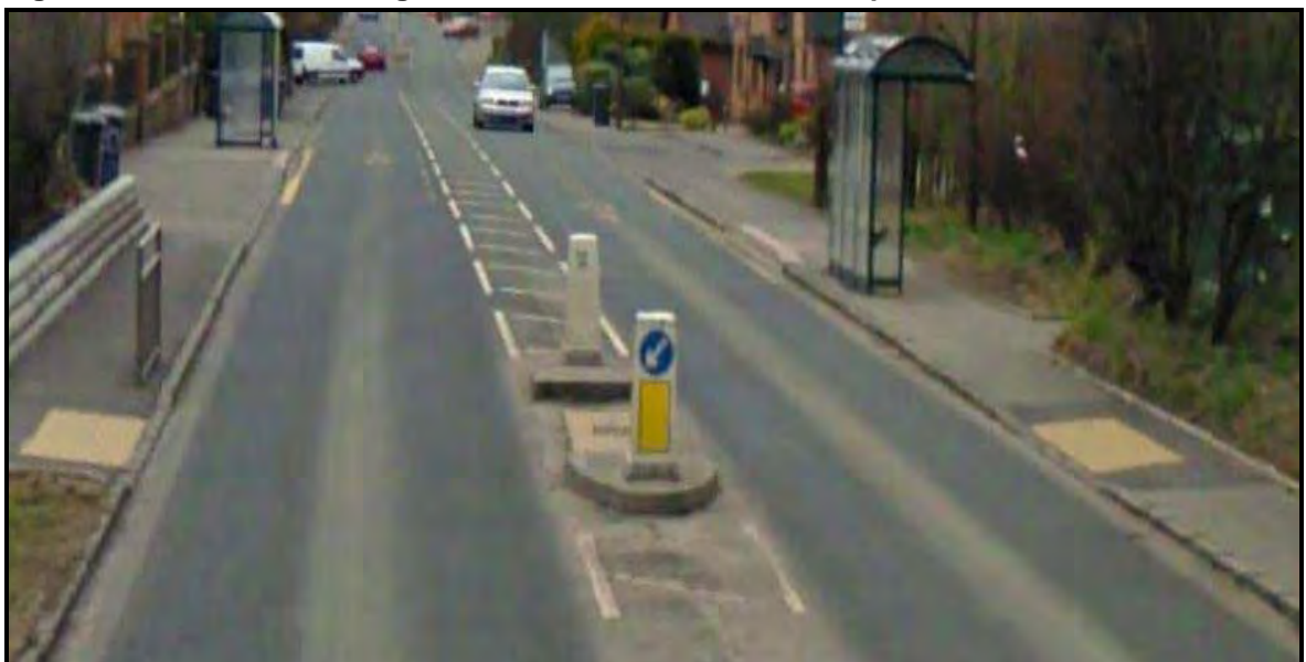
Figure 3.3 Informal Crossing Points to the West of the Development Sites
