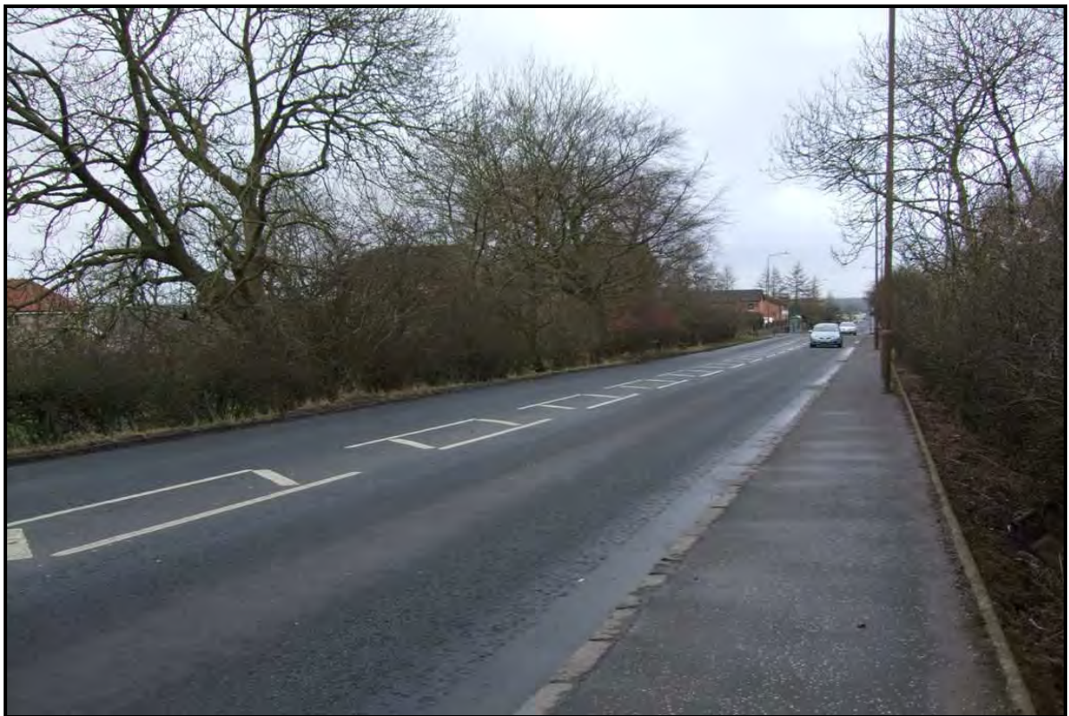
Figure 3.2 Standard of Footway on the A705 Seafield Road
