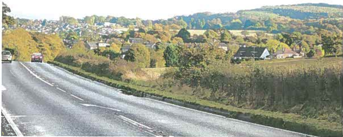
View approaching Linlithgow Bridge on the A803
