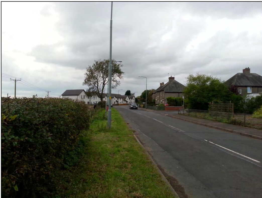
Verge on site side (left of picture) can be used to enable footway connections
