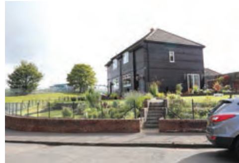
Swedish timber housing - Adjacent to site
