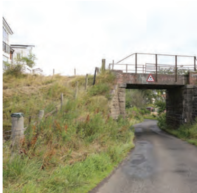
Existing bridge to be removed
