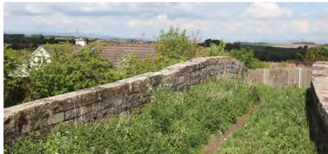
Desire lines over the bridge
