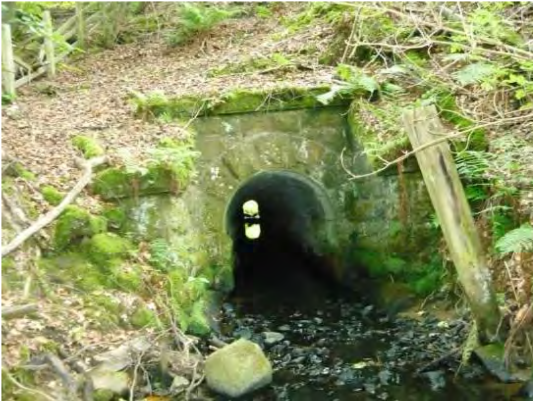
Plate 3: Culvert under Murieston Road
