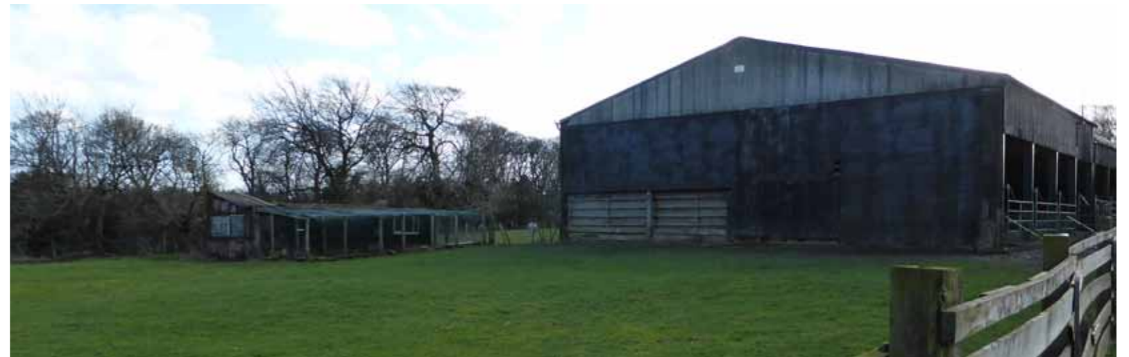
View 10: Brotherton Farm building and treebelt screening proposed site beyond.
