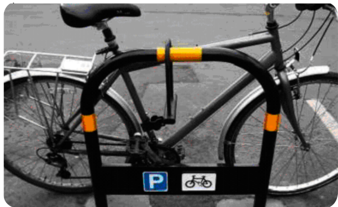
The Sheffield Stand provides good support to the cycle and allows the cyclist to secure both the frame and wheels without risk of damage.
