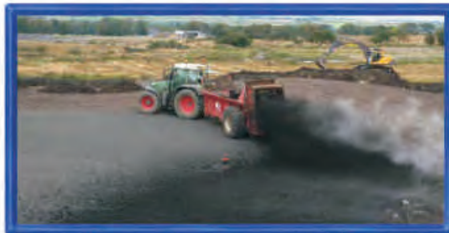
The organic compost is spread over the colliery waste in carefully calculated amounts.
