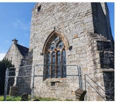
It is recommended that appropriate repair work is undertaken as a priority to repair the masonry of the window frame and to replace missing glass panes and brickwork.
