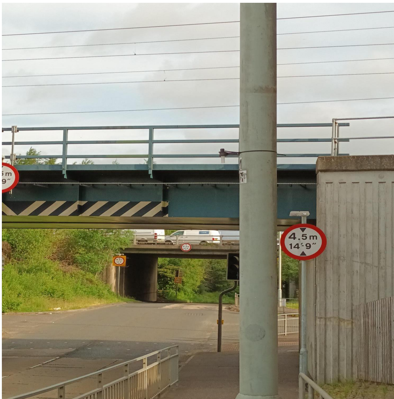
New Diffusion Tube Location – Uphall Station – Installed In September 2022
