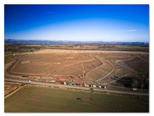
Remediation of the Auldcathie site was zoned based on the findings of earlier investigation, waste delineation during remediation and the proposed end use of the area. The core of the strategy was to provide an engineered landfill cap and gas collection system across the main biodegradable landfill with works area. comprising waste reprofiling and construction of a composite geosynthetic and geological
