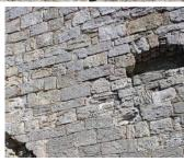
The characteristics on the building façade should be repaired and re-pointed in order to preserve the existing stonework. Repair work will reduce erosion significantly. This will also improve the overall appearance of the historic features.
