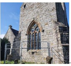
It is recommended that appropriate repair work is undertaken as a priority to repair the masonry of the window frame and to replace missing glass panes and brickwork.
