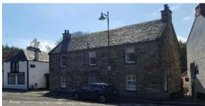
The Gatehouse was built sometime after the church but the same style and materials were used in its construction. The envelope and chimney materials consist of random rubble, and the material used for the skew-gabled roof is slate.
