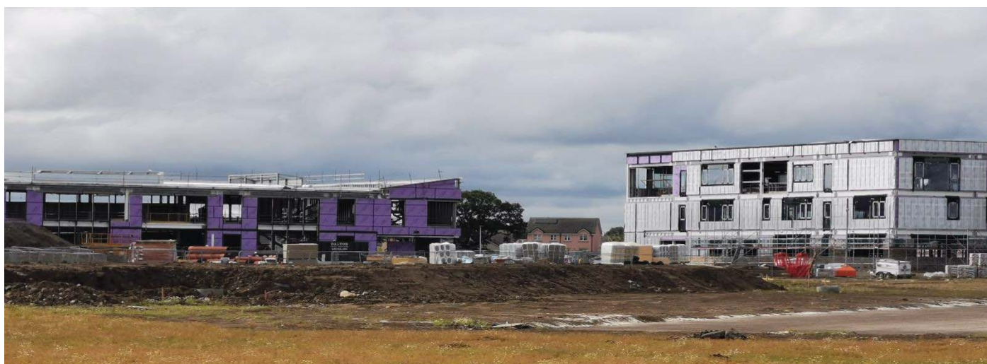
Winchburgh Denominational Primary and Secondary Schools taking shape on site
