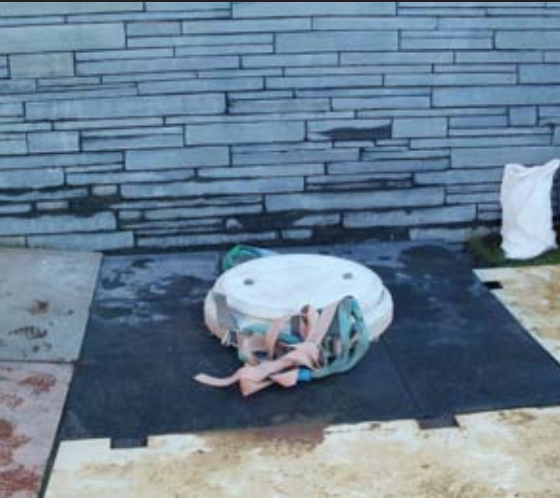
The Base is measured and laid
