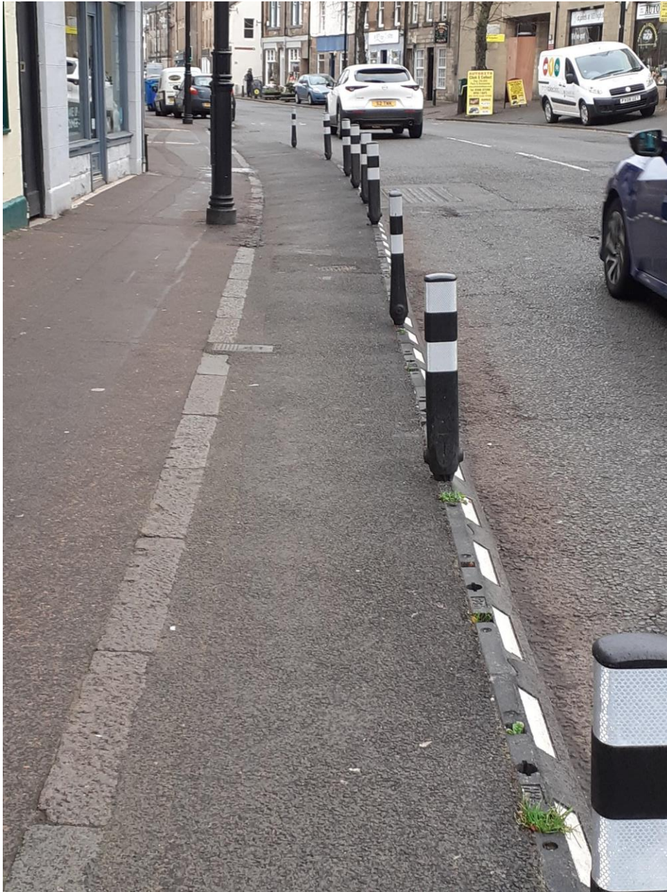
Widening of pavements in Linlithgow during the pandemic to encourage active travel
