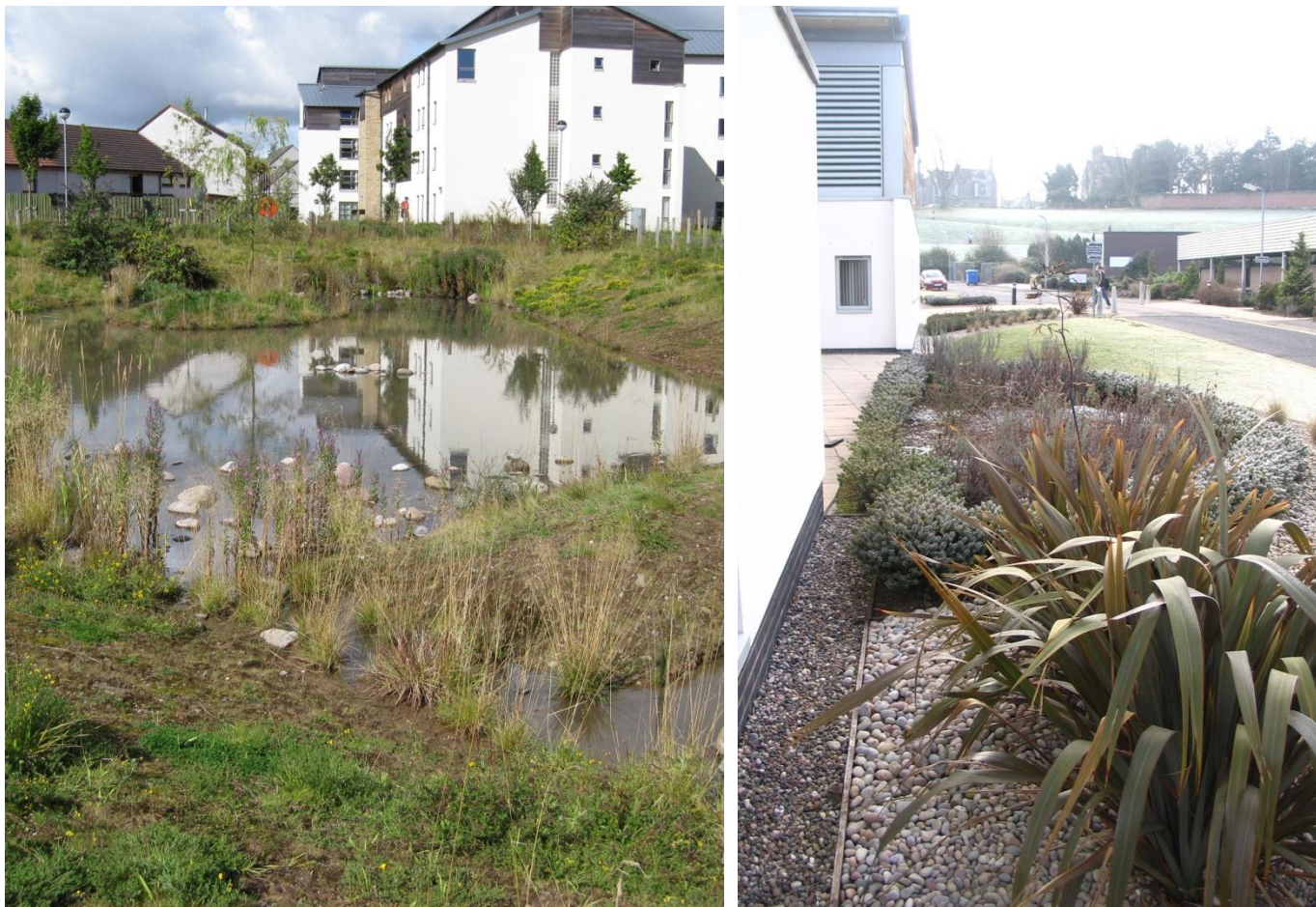
Swales, ponds, trees and permeable surfaces visually enhance hard surfaces and provide benefits to runoff and drainage
