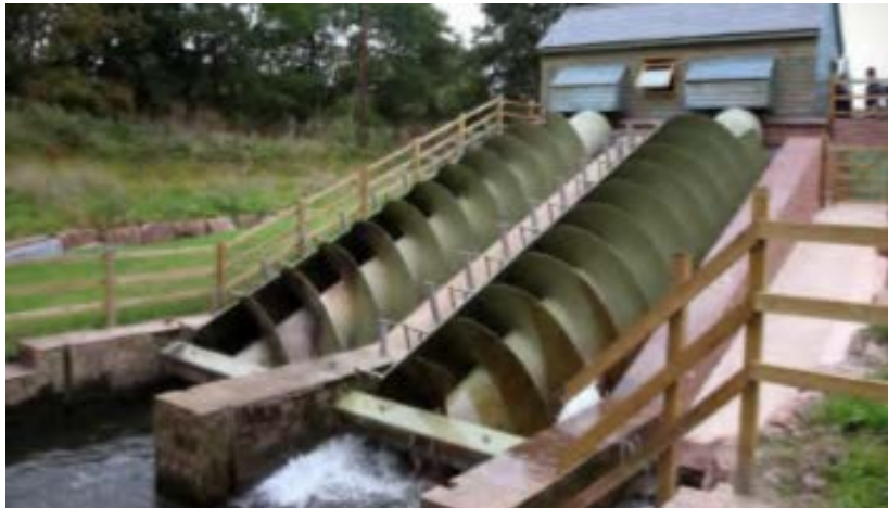
Figure 6: An 'Archimedes' screw diversion
