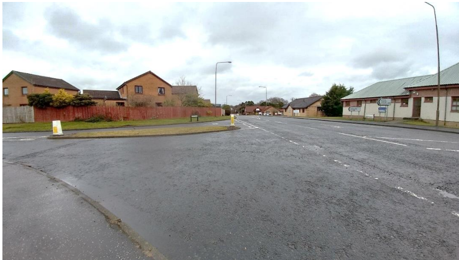
Image 6.36 - Footway Ends at Muirieston West
