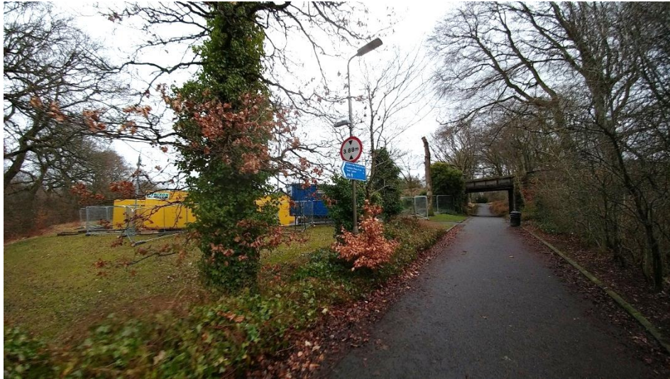
Image 6.50- Bankton Mains Path to the South showing Site Compound
