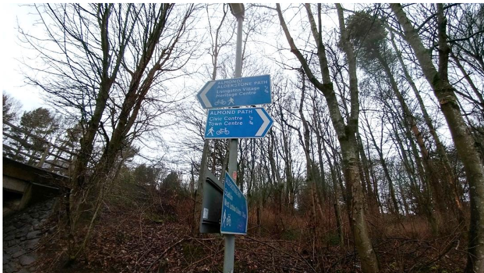
Image 6.23 - Twisted signs on multiple panels
