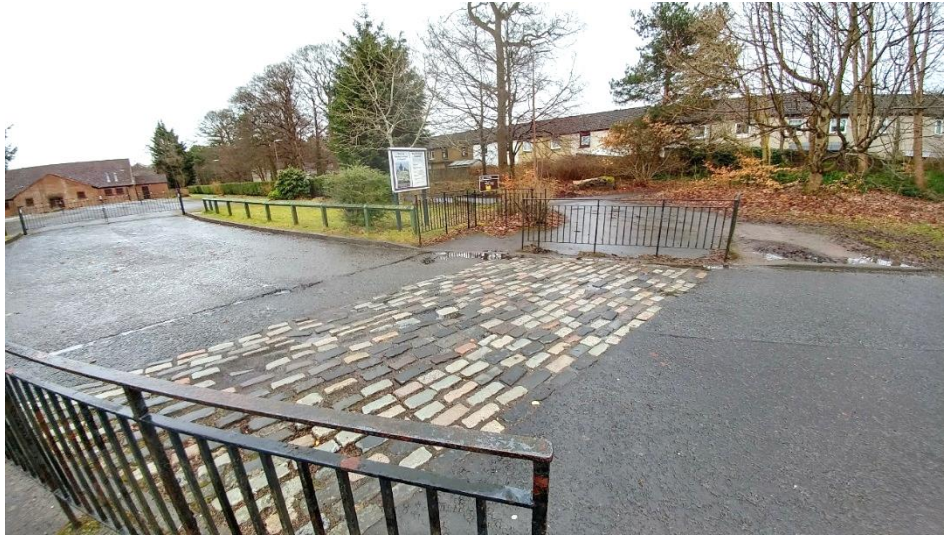
Image 6.10 Lack of clear information on route crossing road
