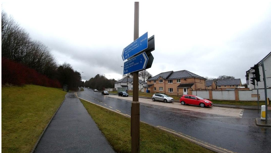
Image 6.25 - Signage at right angles to direction of travel
