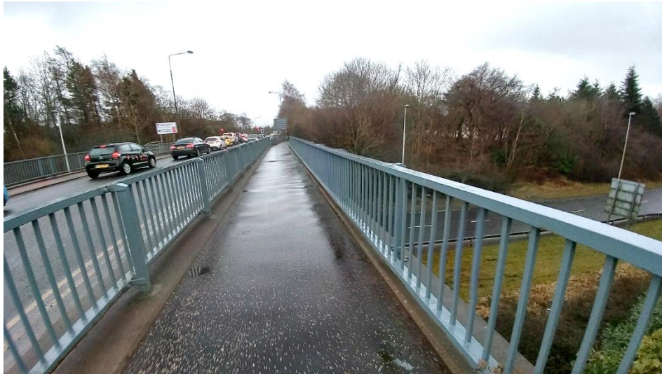
Image 6.14- Bridge with low parapet height
