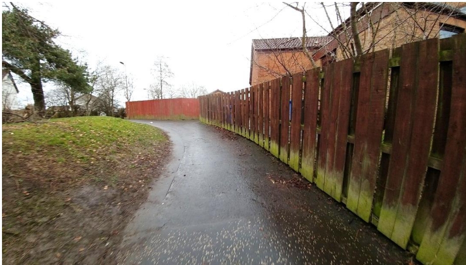
Image 6.44 - Bankton Mains Path after Underpass
