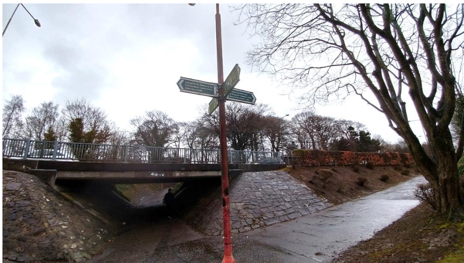
Image 6.13- Difficult to read signage
