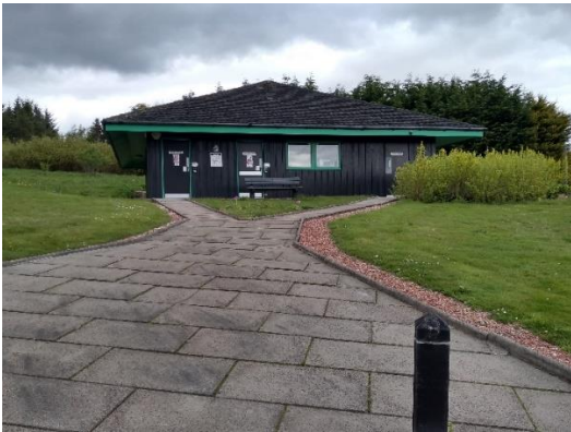
Caravan site ablution block pathway
