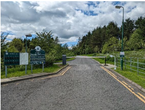
Caravan & camping site entrance, layby and key boxes – use keyfob to gain access
