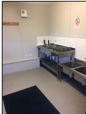
Dishwashing room adjacent to hardstanding pitches
