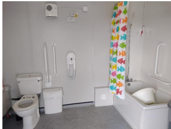
Disabled shower room – caravan block
