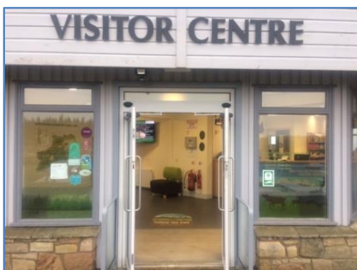
Visitor Centre main entrance & foyer
