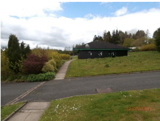
Caravan site pathway from Cherry Hollow to ablution block
