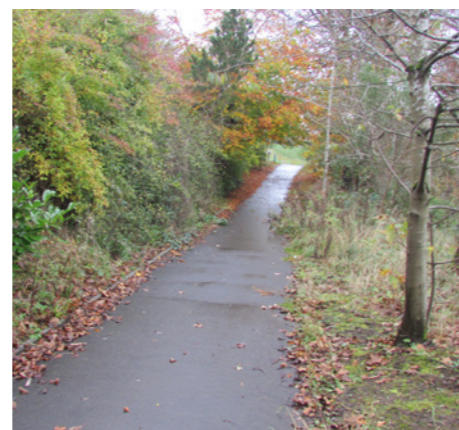
vegetation needs to be cleared along path edges
