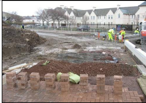
Photo 4. Road Construction Type M1 in Progress
