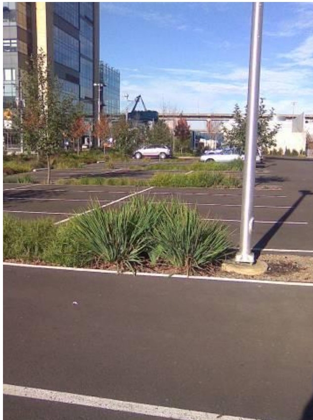
Figure 2.9 Bioretention Cells in Car Park – No Kerbs or Gullies.
