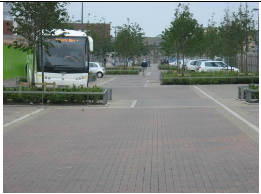
Photo 2. Permeable block paving on the site
