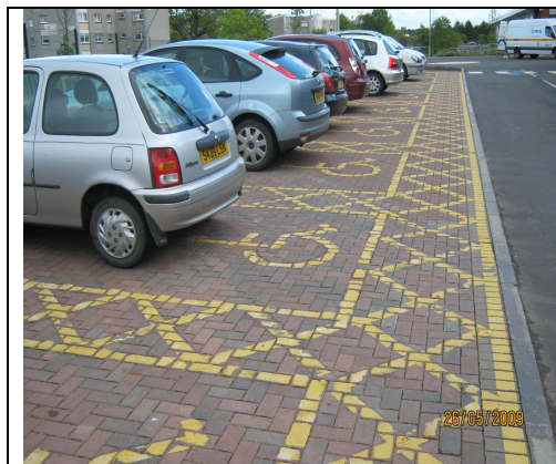
Photo 7. Permeable paving at disabled parking spaces
