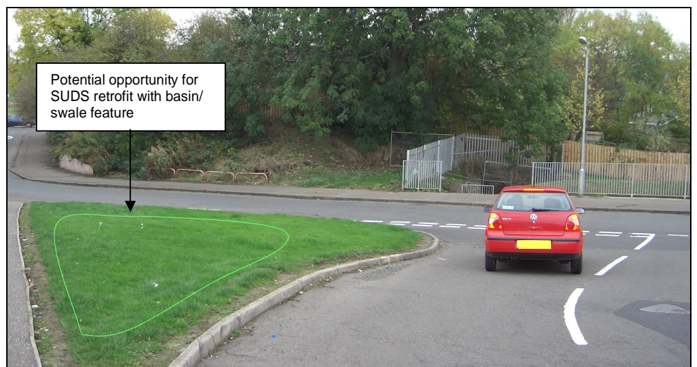
Figure 5.5 SUDS Retrofit at Junction, South Lanarkshire
