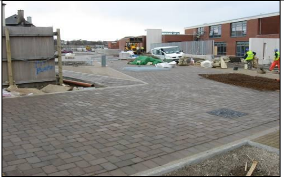
Photo 5. Road Construction Type M2 Completed
