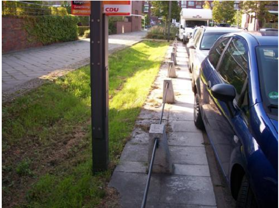
Figure 2.8 Roadside Swale - Flush Kerbing and Low Barrier Keeping Vehicles out of Swale.
