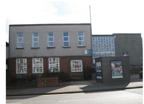
West Lothian Council Building at 'The Cross'
