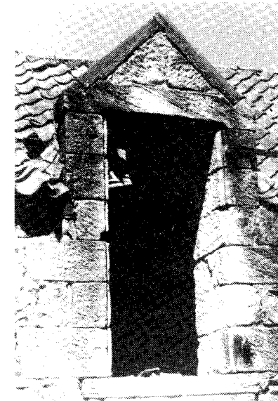
7. South Mains: upper storey boal hole in barn.
