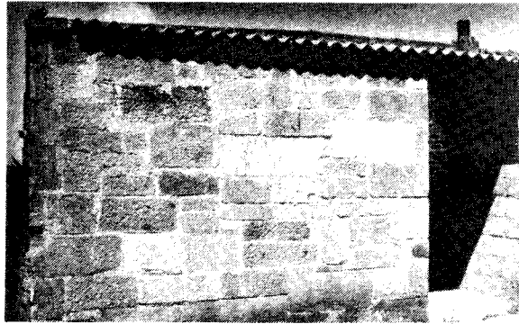
8. Cathlawhill: stable wall constructed of squared sandstone rubble.
