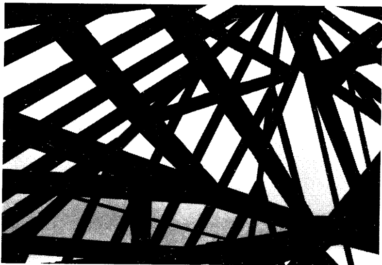
The Byres: Roof of horse mill.
