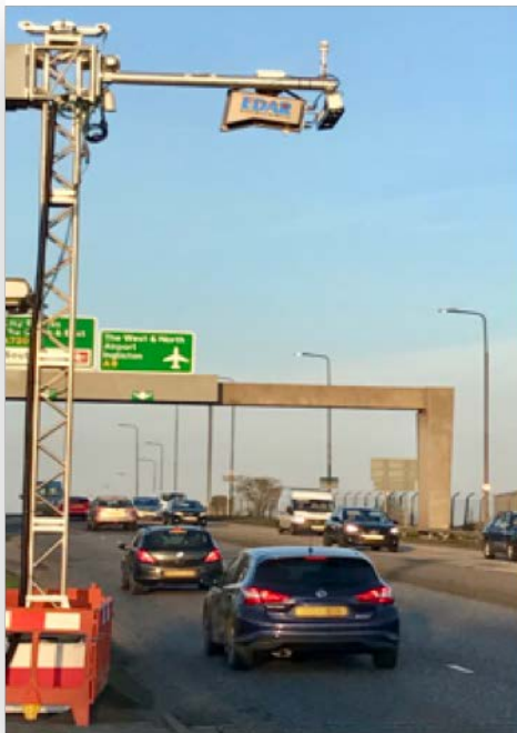
Figure 3-1: Truss System Deployed On Road
