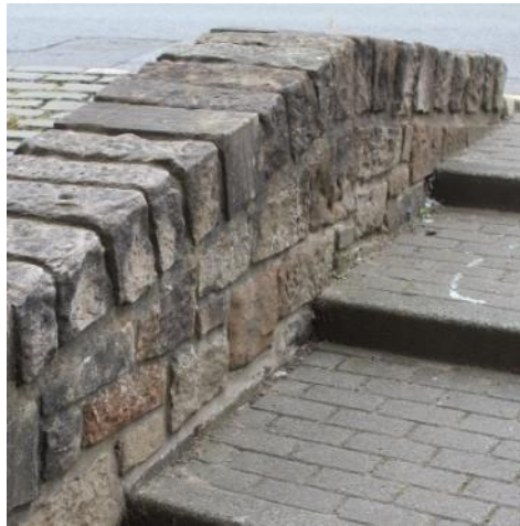
High quality existing stone materials could be reused to resolve levels issues.
