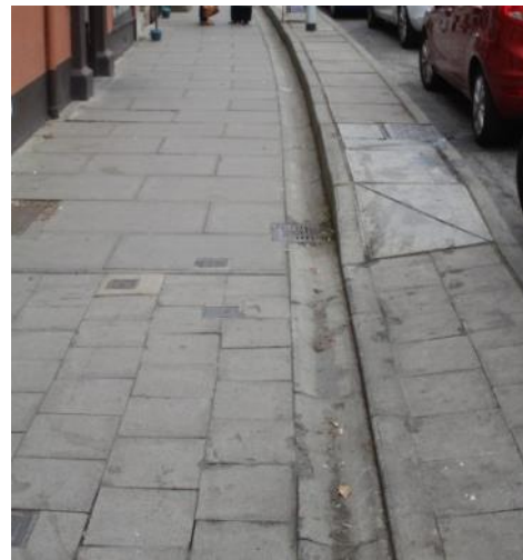
Numerous level changes impede pedestrian flow.
