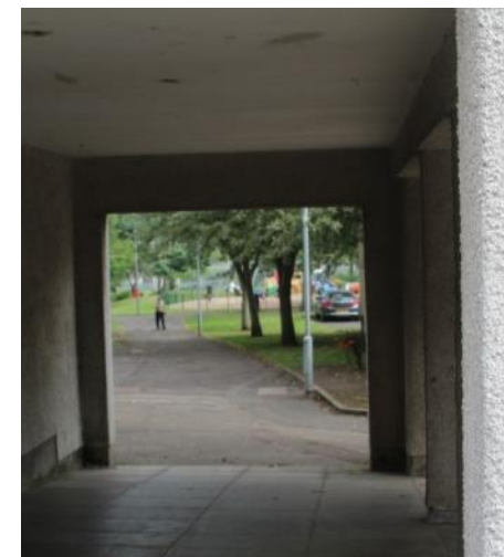
Visual connectivity between the High Street and Lochside Park is restricted. Improving visual linkages and pedestrian routes would promote the town's distinctive water-side setting.
