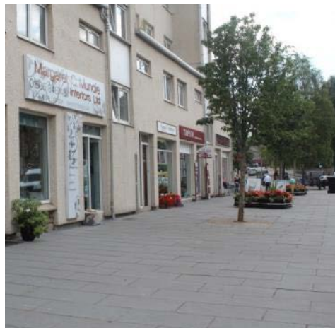
Left: Modern shop frontages and poor street tree planting detract from the High Street.
