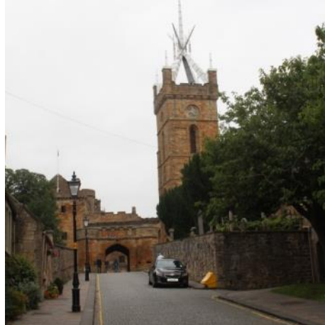
Left: High quality paving leading up to Linlithgow Palace and St Michael's church flanked by high stone walling.
