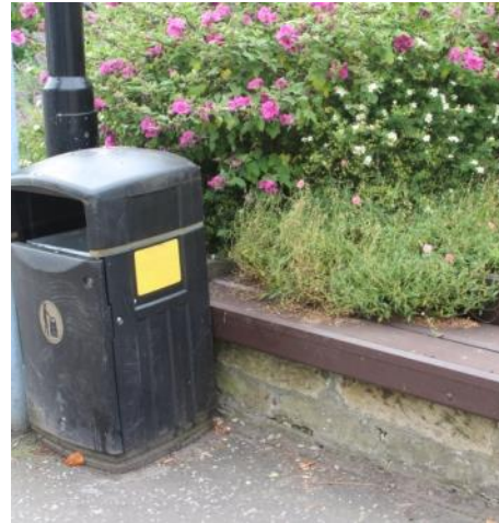
Shrubs encroaching over High Street seating and poorly located litter bin create an unattractive and unusable public realm at St. John's Avenue.
