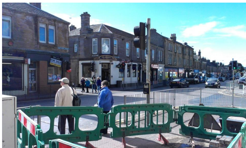
Figure 2: Broxburn site visit
