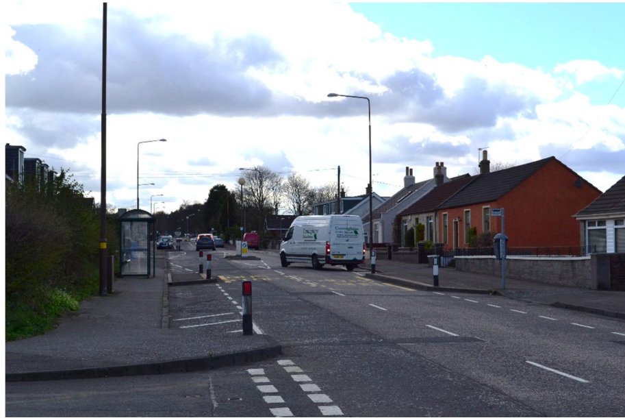
Figure 4.6- Typical view of bus top build out and on street parking.
