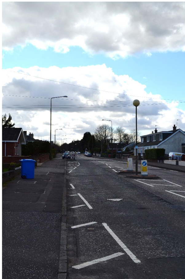
Figure 4.5- Typical view of Main Street.
