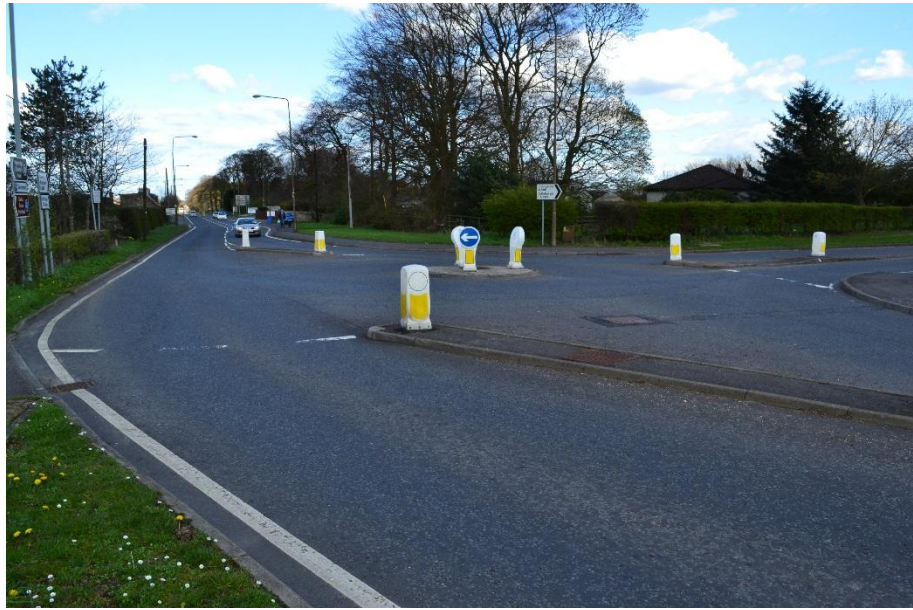
Figure 4.9- Main Street / A899 Mini roundabout.
