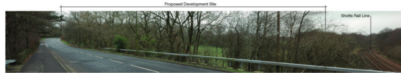
View south-west from railway crossing over Murieston Road with trees screening rail line
