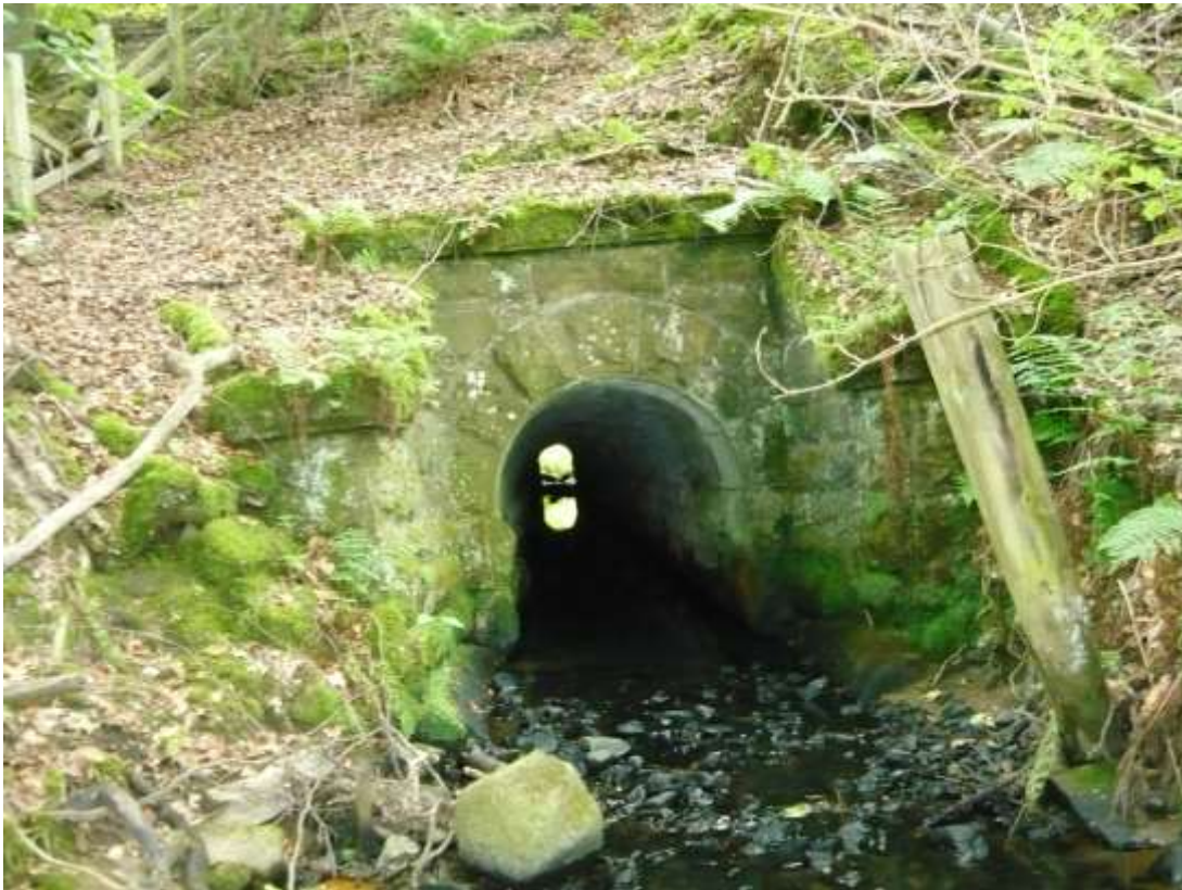
Plate 3: Culvert under Murieston Road
