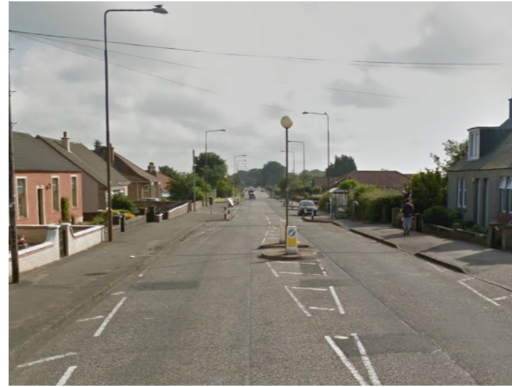
Main Street (eastwards) - broad main street with set-backs
