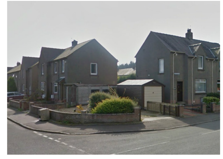
Craiglaw - 2 storey terraces with low-wall block boundaries
