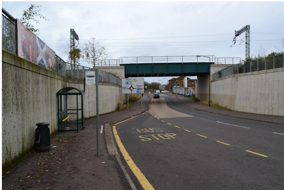
Figure 2.3: Existing bus facilities on Linkston Way.
