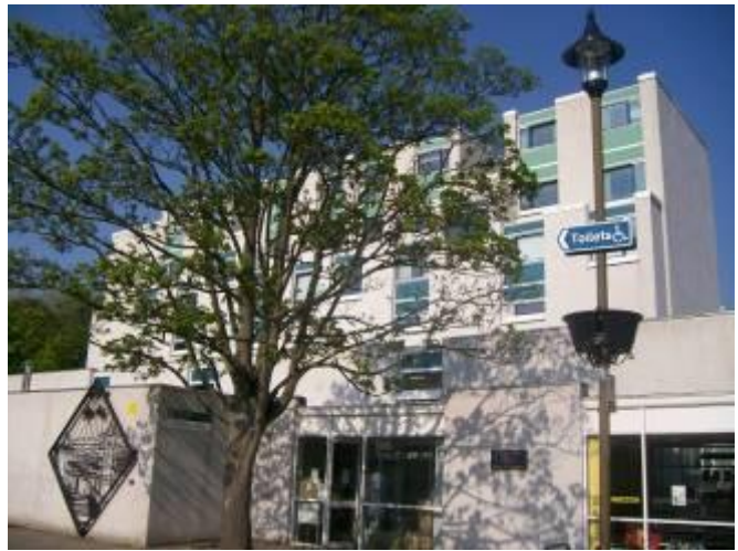
The forthcoming relocation of public library from Guyancourt Vennel to the County Buildings augments the area's potential for specialist retailing.
