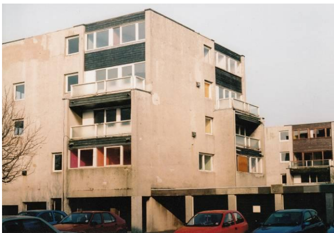
Council flats at St Ninian's Way, demolished in 2002 to make way for private housing.
