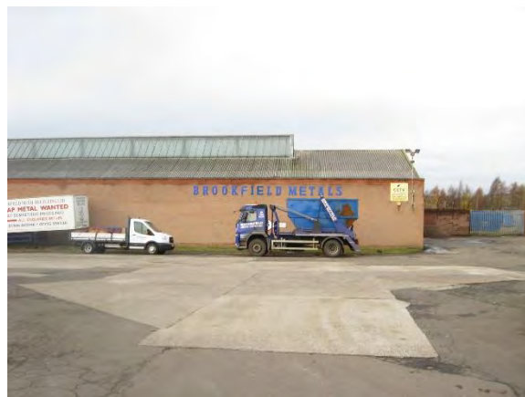
Figure 3: View of Existing Metalworks
