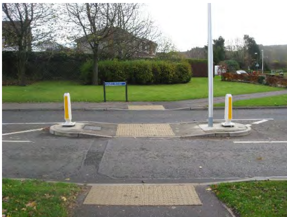
Figure 4: Crossing Facilities Mains Rd (A706)
