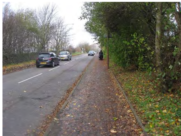
Figure 5: Existing Footway on Mill Road
