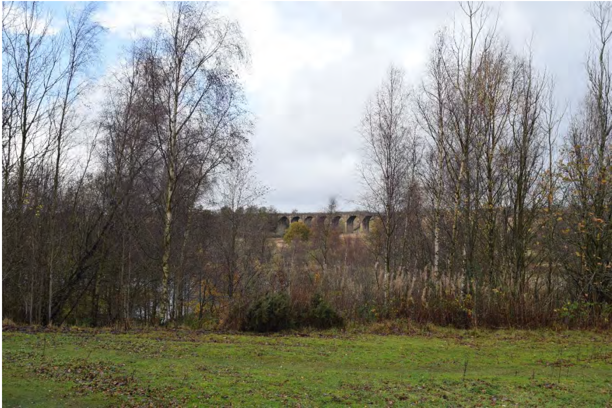
Photograph 7: The Avon Viaduct on the Edinburgh – Glasgow Railway line passes directly to the north of the proposed development site
