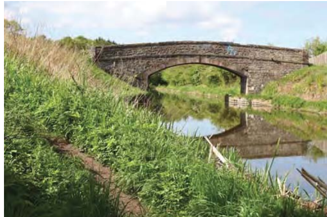
B-Listed bridge connects site to the Union Canal
