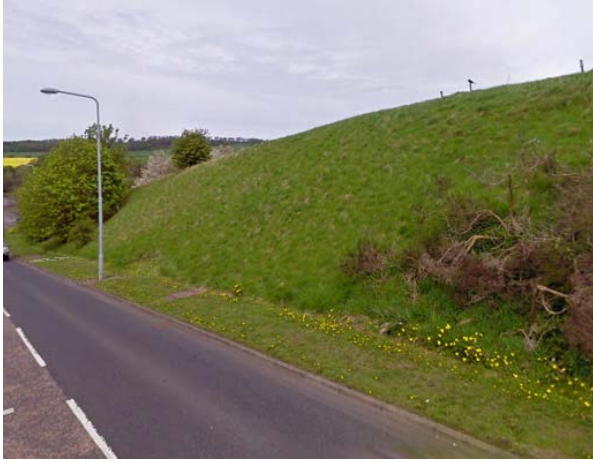
Figure 2 Embankment along Springfield Road
