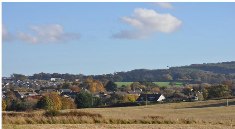
c) HLL-12 is green-buffer introducing Bathgate foothills on Linlithgow's West
