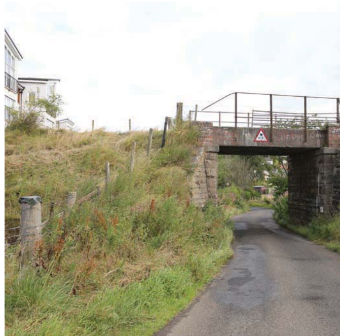
Existing bridge to be removed
