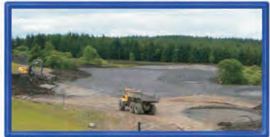
Looking westwards the colliery waste can be seen here layered on the fairway of Hole 4,
