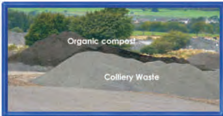
In the 1st project of its kind in the UK the golf courses are being built by combining screened colliery waste shale with locally sourced high-quality green organic compost.
