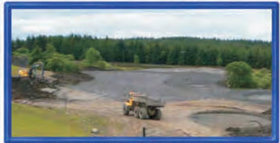
Looking westwards the colliery waste can be seen here layered on the fairway of Hole 4.
