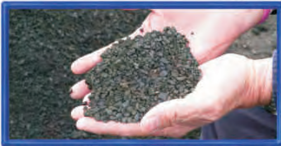
Inert colliery waste has been crushed, screened and graded and is being used as the base for the fairways.
