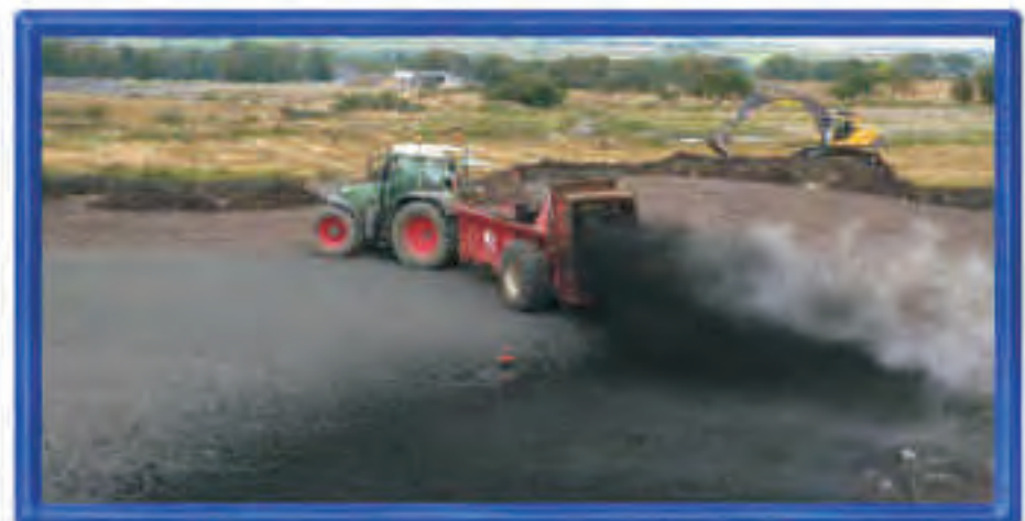
The organic compost is spread over the colliery waste in carefully calculated amounts.
