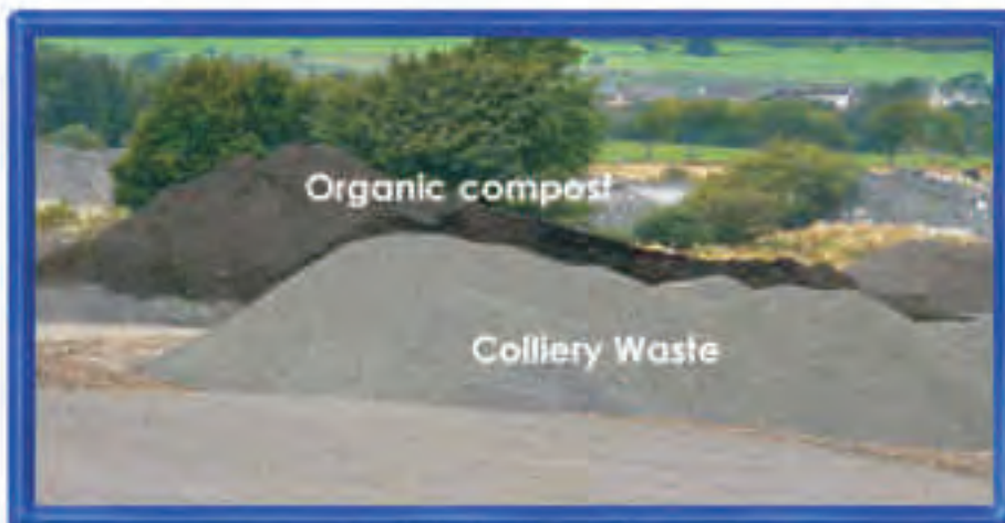
In the 1st project of its kind in the UK the golf courses are being built by combining screened colliery waste shale with locally sourced high-quality green organic compost.
